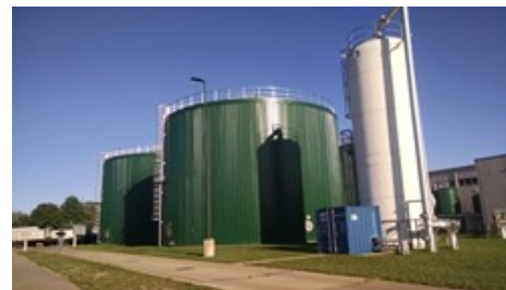
| Fremont Regional Digester
