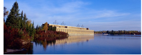
Slave Falls Generating Station | Manitoba Hydro
